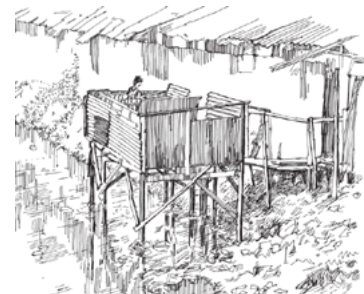
Figure 31. Hanging toilet/hanging latrine
